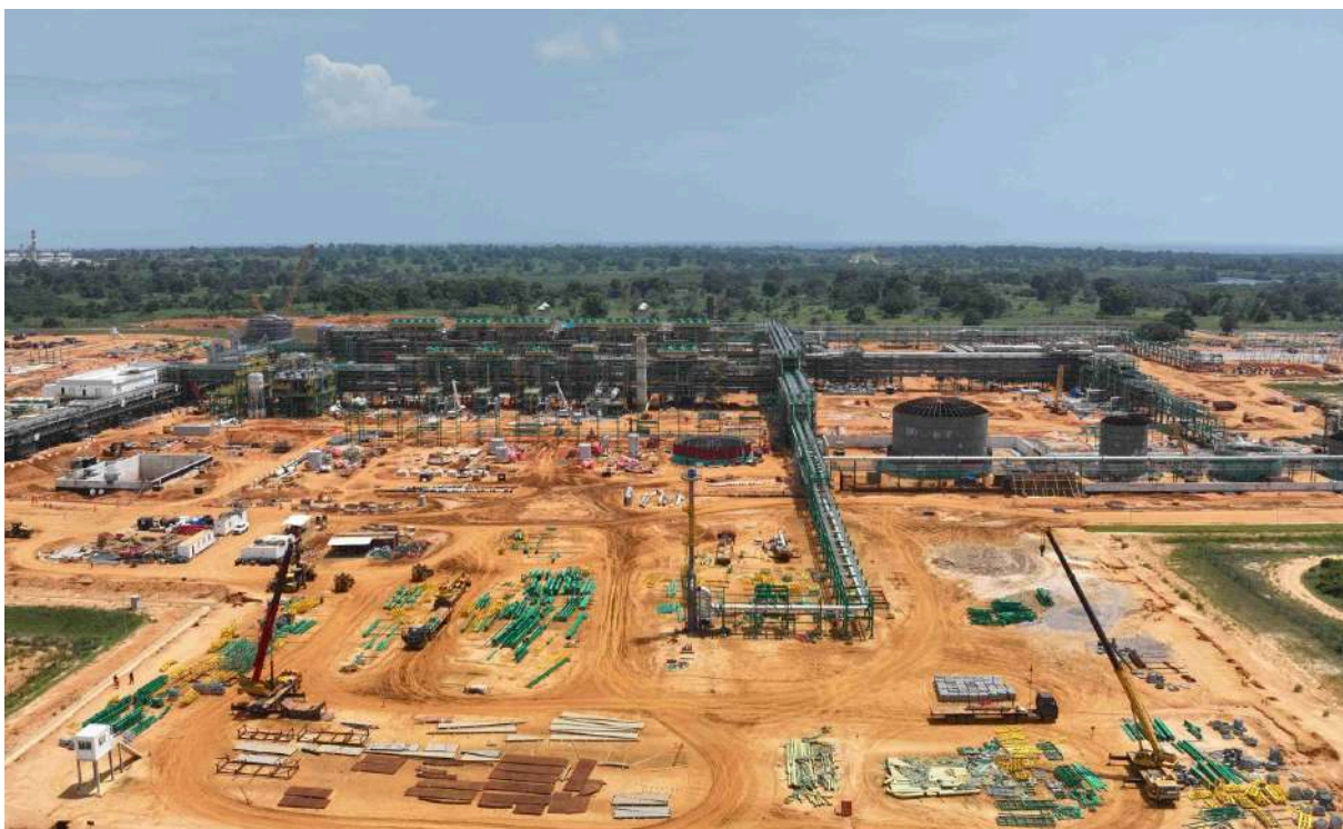
Projeto Oil & Gas, Quiluma & Maboqueiro Project (Saipem) - Soyo, Angola Oil & Gas Project, Quiluma & Maboqueiro Project (Saipem) - Soyo, Angola
