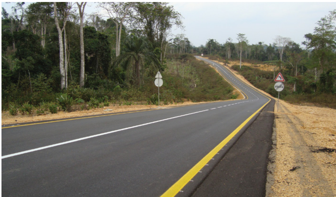
Estrada Buco Zau – Sanga Mongo (28 Km), Cabinda. Cliente: INEA – Ministério da Construção. Route Buco Zau – Sanga Mongo (28 Km), Cabinda. Client: INEA – Ministère de la Construction. Buco Zau Road – Sanga Mongo (28 Km), Cabinda. Client: INEA – Ministry of Construction.
