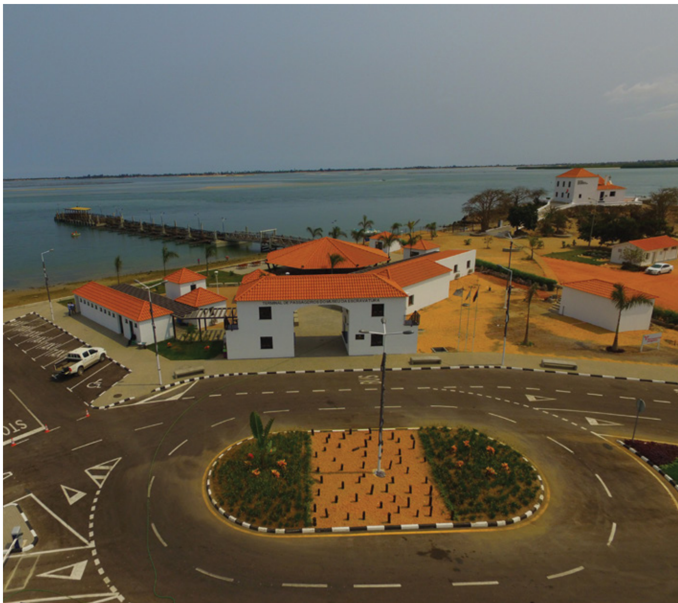
Construção do Terminal Marítimo de Passageiros do Museu da Escravatura, Luanda. Cliente: IMPA – Ministério dos Transportes. Construction du Terminal Maritime de Voyageurs du Musée de l'Esclavage, Luanda. Client: IMPA – Ministère des Transports. Construction of the Passengers Maritime Terminal of the Museum of Slavery, Luanda. Client: IMPA – Ministry of Transport.
