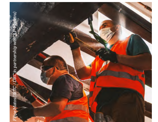
Requalification of the Church and Convent of Santa Clara, a 15th century national monument, an ongoing project in Funchal
