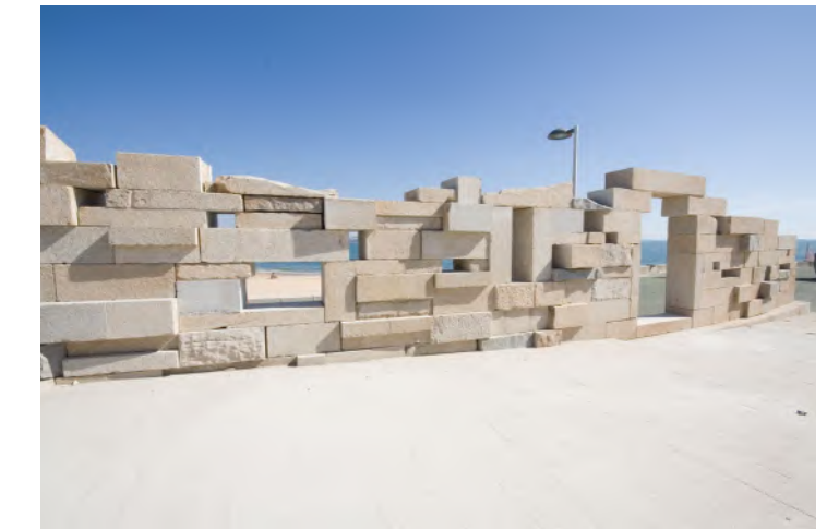
Built by Tecnovia in 2009, Passeio Marítimo de Oeiras – Paço de Arcos is one of the most used leisure spaces in the municipality
