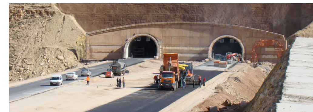
Zaouiat Ait Mellal, a double gallery road tunnel integrated in the construction a section of 13 km of the Chichaoua-Argana Highway, Morocco, built by Tecnovia in 2009
